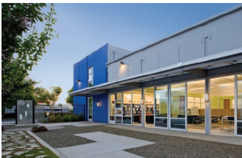
IDeAs Z2 Office Renovation, San Jose, EHDD The Z2 (zero energy zero carbon) office design turned a windowless 1960s bank building into a high-performance daylight office building for the electrical engineering firm IDeAs (Integrated Design Associates, Inc.). Photo by David Wakely.
