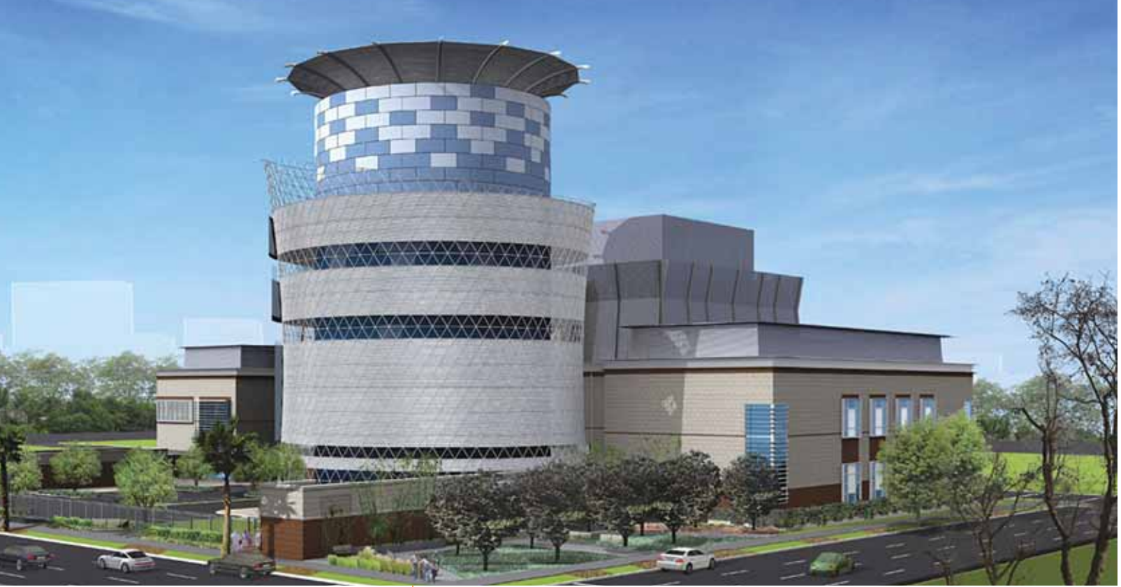
State of California Central Utility Plant, rendering courtesy of Nacht & Lewis.
